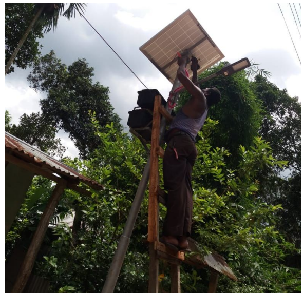
Solar lighting system being installed in Hrishyamukh RD Bloc under RURBAN
